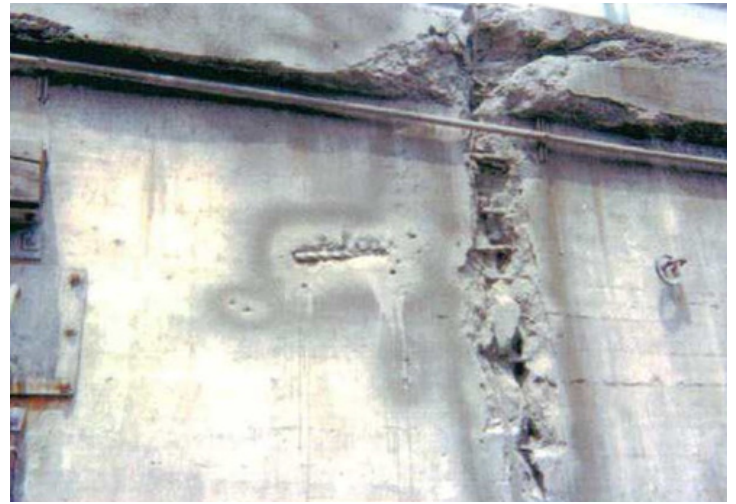
BELOW (left): Dilapidated seawall, with exposed and rusting rebar ; BELOW (right): Corrosion testing being completed on seawall concrete.
