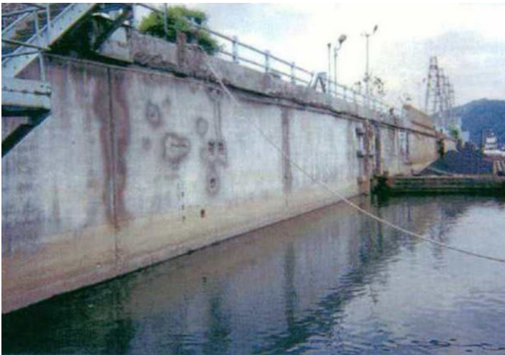
BELOW (left): Dilapidated seawall, with exposed and rusting rebar ; BELOW (right): Corrosion testing being completed on seawall concrete.
