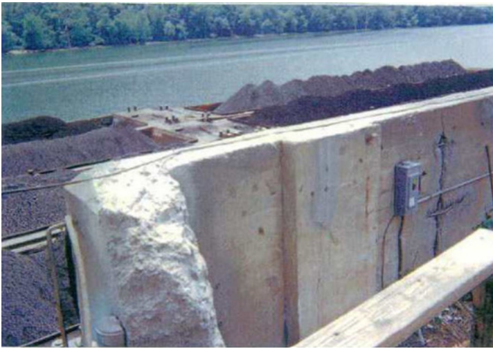
ABOVE: Dilapidated seawall, with exposed and rusting rebar.
