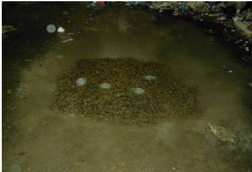
Figure 2: Overview of treated and untreated tipping floor areas cored
