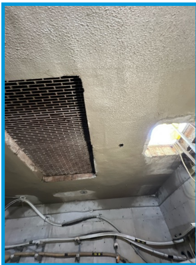
PICTURED: Completed Vault
