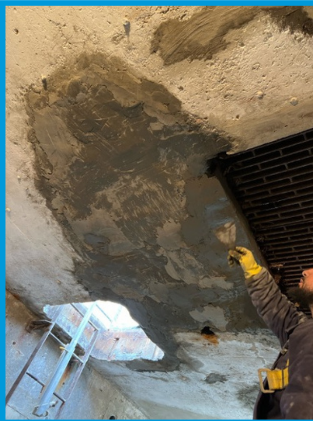
PICTURED (LEFT): After application of FRP Primer
