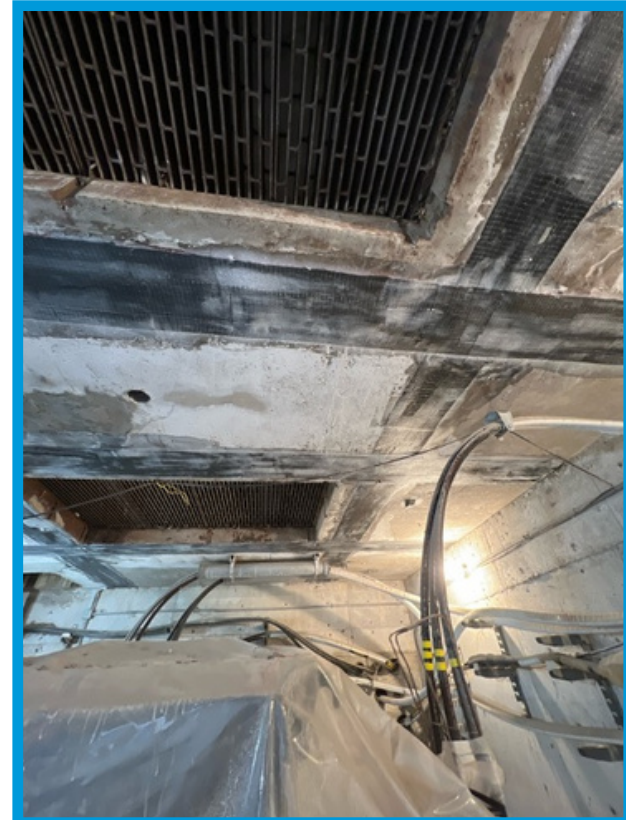
PICTURED (RIGHT): CFRP Installation
