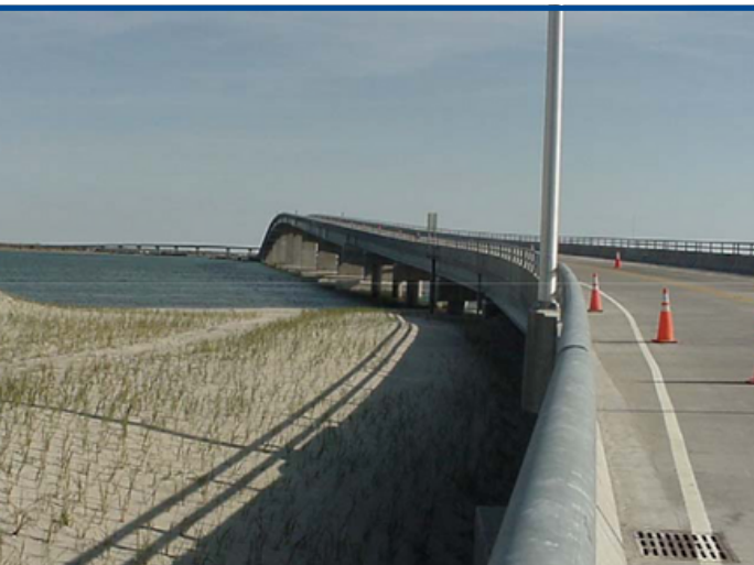
LEFT: The Ocean City Longport Bridge
