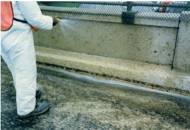
LEFT: Surtreat being applied to bridge.
