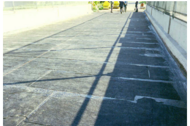
RIGHT: Permaquik water proofing system applied..
